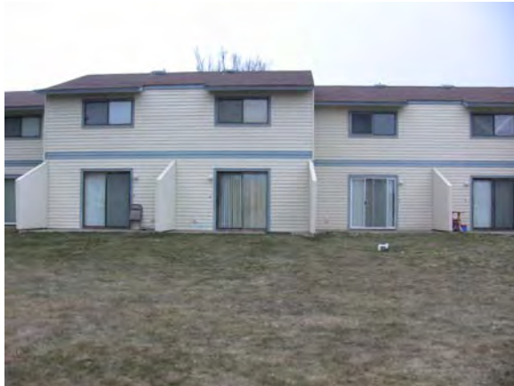
Back of Building-Patios
