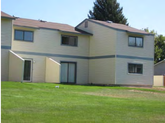
Back of Building D
