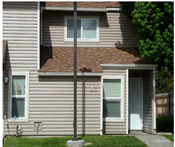
Front of Building A
