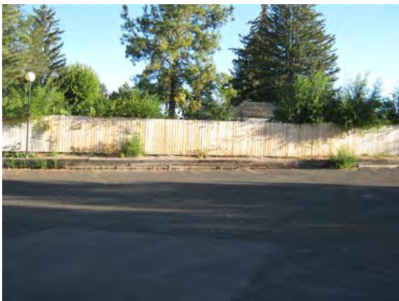
Railroad Tie Retaining Wall
