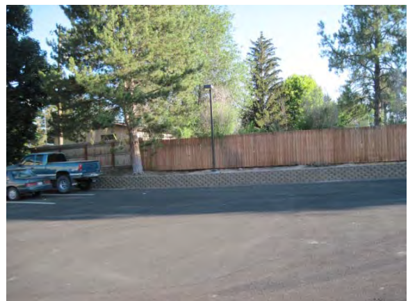
New Keystone Wall
