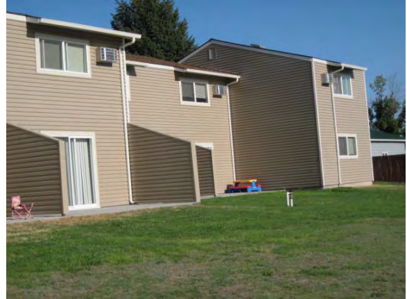
Back of Building D
