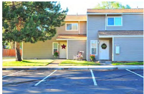
Front of Building B
