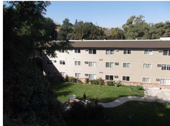
Side of Building with Gazebo Removed
