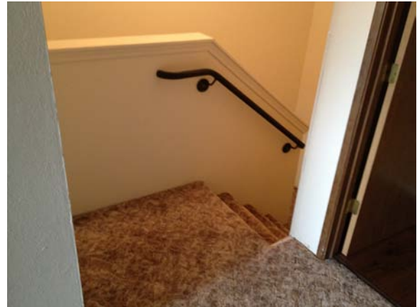
New safety wall at Unit Stairs
