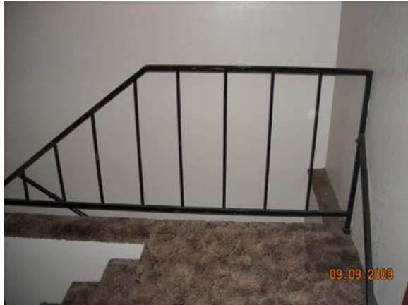
Handrail at Unit Stairs
