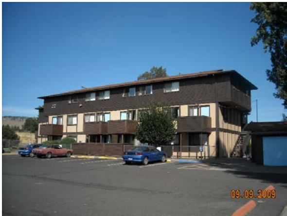
Back of Building 6
