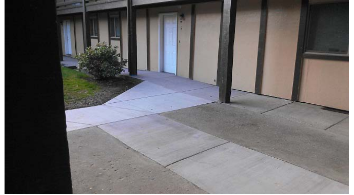
Western Complex Courtyard New Accessible Route
