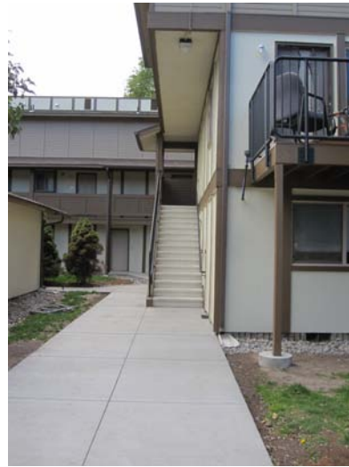
Side of Building 2 Stairs Code Compliant
