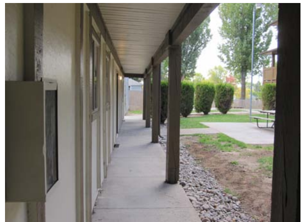
Front of Building 7 New Drainage Installed and Chain Fence Removed
