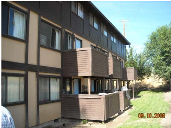
Back of Building 7
