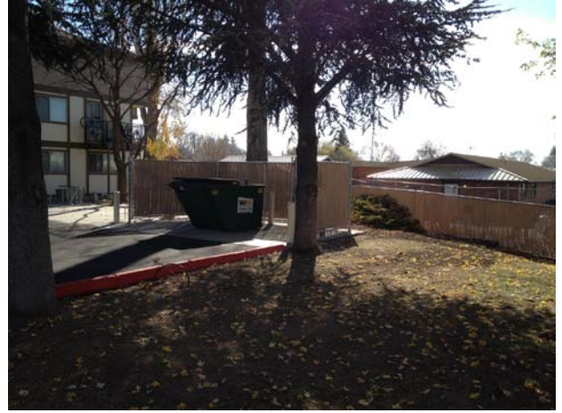
New Trash Enclosure
