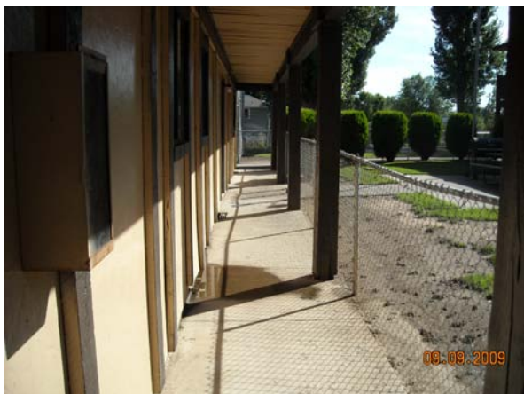
Front of Building 7
