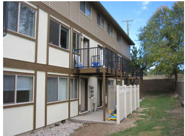
Back of Building 7
