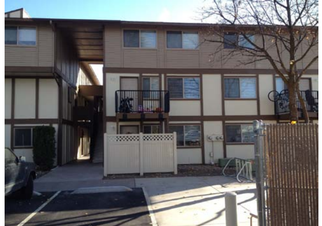
Back of Building 1
