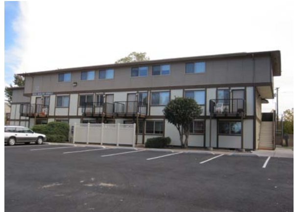
Back of Building 6
