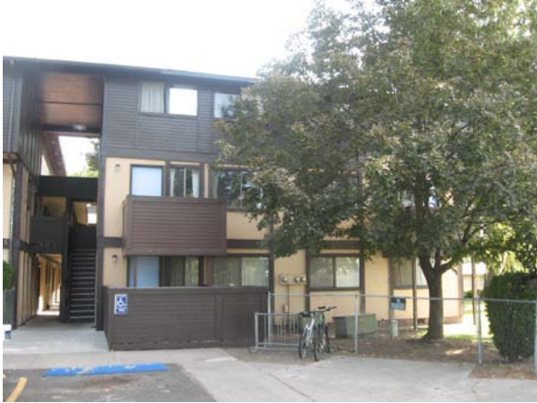
Back of Building 1
