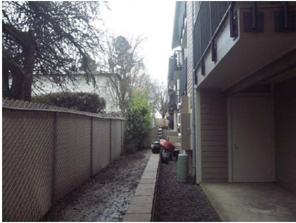
Fencing Behind Building with New Keystone Block Wall
