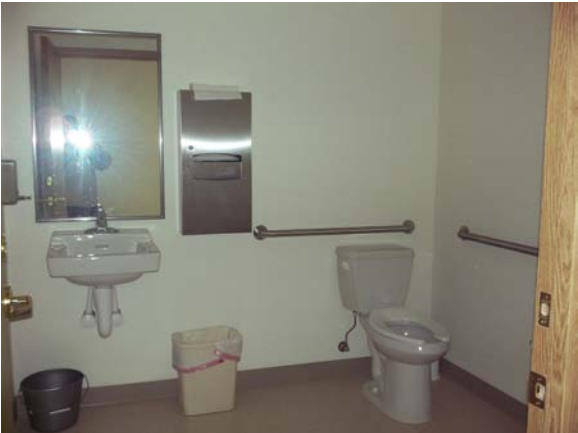
New ADA Restroom in Laundry Room
