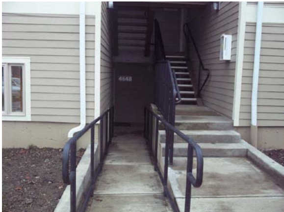
New Ramp with Railings
