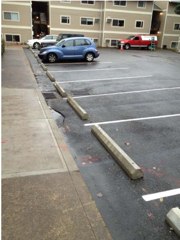
Striping and New Wheel Stops in Parking Lot
