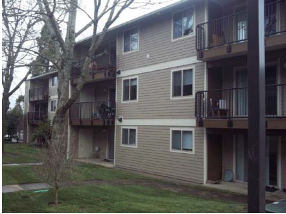
Balconies with new Railing, and New Windows
