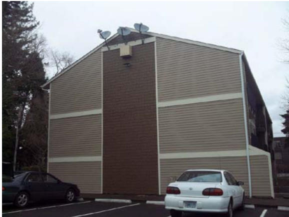
Siding on Building
