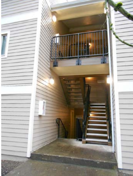
Stairwell with new Lighting and Railings
