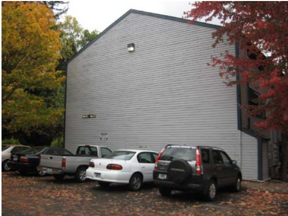
Siding on Building
