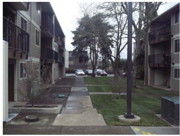
Courtyard with new landscaping and site lighting
